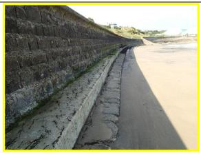
Erosion and spalling of front face of wall. Asset Ref. 1221D901D1201C03
