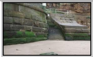
Photo from 2009 showing repairs visible, voids and gaps (Asset Ref. 1221D901D0802C12)
