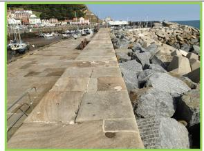
East Pier rock armour and Accropodes showing area of possible settlement of crest armour (Asset Ref. 1221D901D1301C01)
