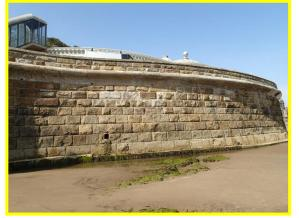
Repaired splash beam, but cracks in blockwork below (Asset Ref. 1221D901D1301C28)
