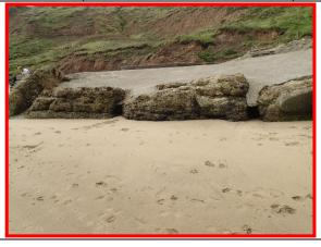
Around 300m south there is a beach access point for the path from the public car park at the surf shop. There are a set of beach access steps that were previously protected by gabion baskets, which have distorted and split under wave action and / or cliff movement, see below left and right. This is not a formal coastal defence, so has no asset number.
