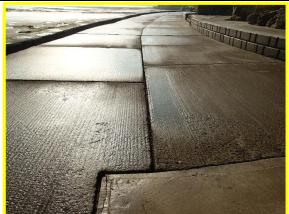
Missing joint sealant in gaps promenade slabs (Asset Ref. 1221D901D1303C02)
