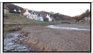
Low masonry wall at East Row Beck, south bank, Photo from 17th December 2013. Note accumulation of sand with the beck cutting through. (Asset Ref. 1221D901D0702C03)
