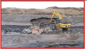
Temporary repairs to revetment being carried out on **17th December 2013**. (Asset Ref. 1221D901D0702C02)
