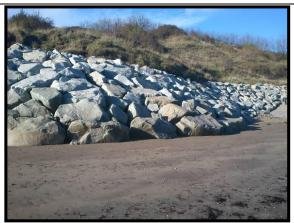
Tightly packed rock armour in good condition in 2012– **photo from 2012**(Asset Ref. 1221D901D1003C07)
