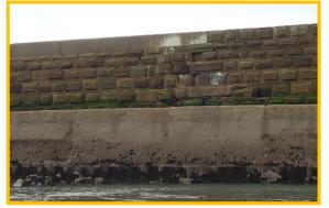
Example area of displaced blocks on outer (W) face of East Pier (Asset Ref. 1221D901D0803C03)
