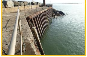
Corrosion of sheet piling on the landward side of the north breakwater (12/09/2014) (Asset Ref. 1221D901D0402C01/4)
