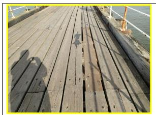
Damage to ends of timber desk on West Pier extension and replacement plank (Asset Ref. 1221D901D0803C01)
