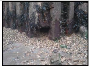
Void under SE corner of breakwater by lighthouse
