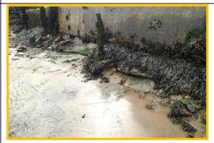
Undercutting at the toe of some parts of the harbour wall (no change since 2009) (Asset Ref. 11221D901D0402C22)
