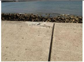
Previous minor repair to crest wall damage in need of further repair (Asset Ref. 1221D901D1202C02)
