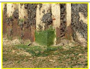
Repair to void under SE corner of breakwater by lighthouse **photo 10/09/2014** (Asset Ref. 1221D901D1301C17)
