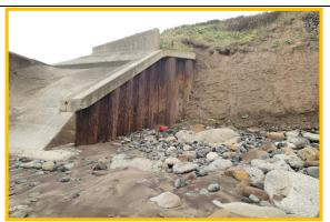
Corroded sheet piling and ongoing erosion at northern end of Sandsend revetment. (Asset Ref No.1221D901D0701C02)
