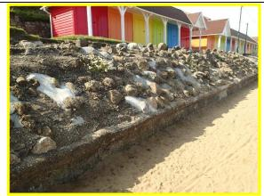
Recent repairs to grouted revetment at rear of promenade. (Asset Ref. 1221D901D1201C05)
