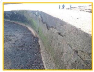
Large horizontal crack to breakwater photo from 2012. (Asset Ref. 1221D901D0601C02)
