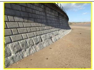
View of wall looking north from near Crescent Hill access, showing abraded lower facing blocks.
