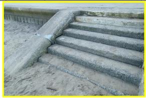
Abrasion damage rounding steps and washout of joints. Asset Ref. 1221D901D1201C17
