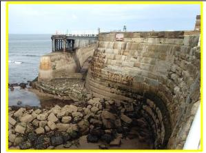
Undermining of apron between main and outer West Breakwater (Asset Ref. 1221D901D0803C02 / 01)
