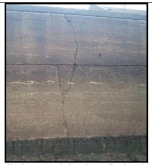
No change to vertical crack extending through the wall **photo from 16/10/12**, with low beach exposing timber toe piles. (Asset Ref. 1221D901D1301C19)
