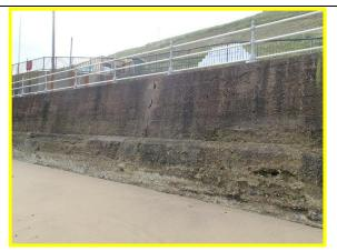
Horizontal and vertical cracks and loss of facing (Asset Ref. 1221D901D0802C04)
