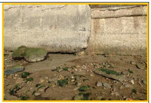
No change since 2009 to undercutting at landward facing of north breakwater (12/09/2014) (Asset Ref. 1221D901D0402C01)
