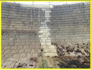
Repair to vertical crack and capping beam north of the ramp. (Asset Ref. 1221D901D1201C21)
