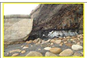
Erosion of cliff adjacent to north end of seawall, 12/09/2014 (Asset Ref. 1221D901D0601C01)
