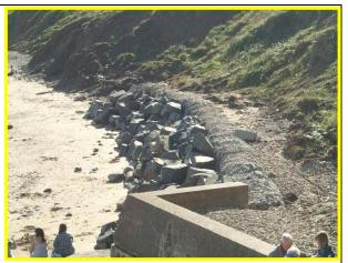
General view of rock armour at interface with natural cliff showing repaired or replaced gabions and re-profiled rock armour, which is again showing signs of displacement.
