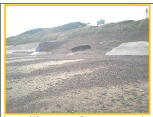
Large void in revetment adjacent to recent patch repair (Asset Ref. 1221D901D0702C02)
