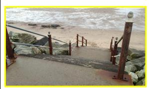
Corroded standards to handrails at steps (Asset Ref. 1221D901D0801C01)
