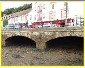
Spalling concrete capping to arched suspended quay at east end of Sandside (Asset Ref. 1221D901D1301C05)
