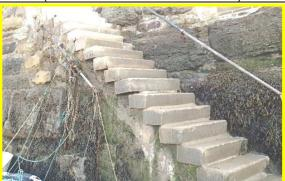
Steps have been repaired, but mortar is starting to wash out again.
