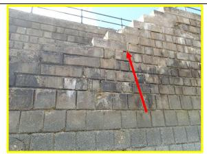
Cracking and open joints between blocks at southern set of steps. (Asset Ref. 1221D901D1602C07)
