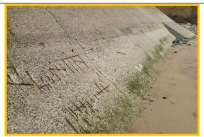
Abrasion damage to revetment exposing reinforcement. (Asset Ref No.1221D901D0701C02)
