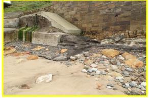
Joint washout abrasion damage and undermining at toe. (Asset Ref. 1221D901D0802C06)
