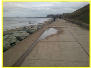
Promenade looking south east showing cracks in slabs and standing water **Photo from 2012** (Asset Ref. 1221D901D0801C01)
