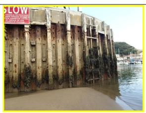
Corroded sheet piling and damaged timber fenders at end of West Pier (Asset Ref. 1221D901D1301C18)
