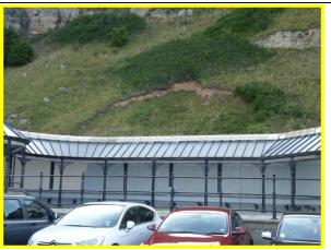
**MU21/2** Talus failure in lower slope (Locally Active). August 2014.
