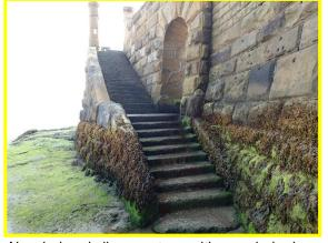
Abraded and slippery steps with rounded edges makes beach access hazardous.
