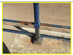
Badly corroded handrails at repaired section of coping. (Asset Ref. 1221D901D1602C03)
