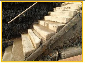
Cracked and loose steps with washed out joints require attention.
