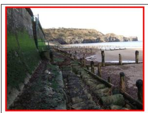
Timber toe of sea wall in a poor state - **photo** from 2009 (Asset Ref. 1221D901D0702C01)
