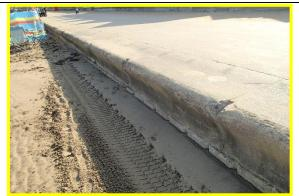
High beach levels in front of beach huts. Minor damage to capping. (Asset Ref. 1221D901D1201C12)
