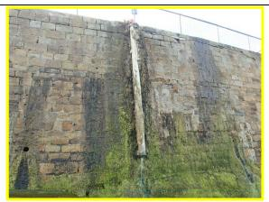
Cracking, mortar loss and vegetation growth due to leaking pipe (Asset Ref. 1221D901D0802C06)
