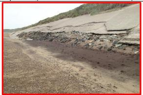
Typical photo of repaired revetment adjacent to previous patch repairs, 12th September 2014. (Asset Ref. 1221D901D0702C02)
