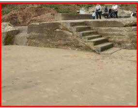
Repairs have been undertaken to patch up the defence at beach access south of the pumping station. (Asset Ref. 1221D901D1402C06)
