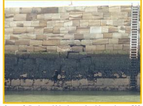
Area of displaced blocks and voids on inner (W) face of East Pier (Asset Ref. 1221D901D0803C03)
