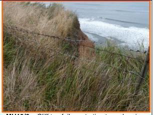
**MU13/6** - Cliff top failure starting to undermine fence – grid reference 492483 510474. August 2014.
