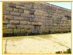
Loose blocks set back in void at toe of wall and open joints (Asset Ref. 1221D901D1301C27)
