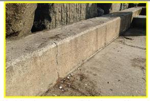
North breakwater crest wall showing cracking and damage from rock movement. (Asset Ref. 1221D901D0402C01)
