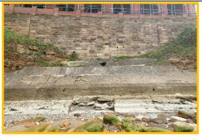
Damage to toe protection and weathering of natural rock below upper wall (Asset Ref. 1221D901D0802C15)
