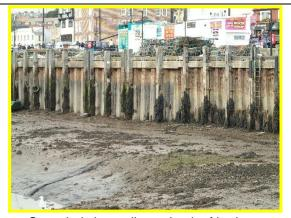
Corroded sheet piles at back of harbour (Asset Ref. 1221D901D1301C12)
