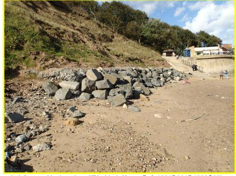
Gabion and rock defence with slumping cliff behind. (Asset Ref. 1221D901D1602C02)
