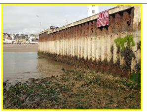
Corroded sheet piles, but overall fair condition
