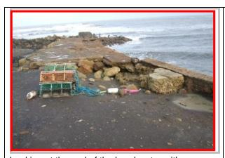
Looking at the end of the breakwater with evidence of erosion and failure in 2009 (Asset Ref. 1221D901D0502C01)
