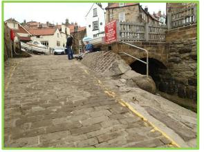
Some loss of mortar in slipway joints, with evidence of multiple previous repairs. (Asset Ref. 1221D901D1003C05)
