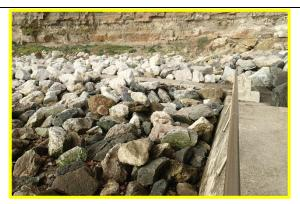
Area of displaced armour stones near root of north breakwater
