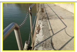
North breakwater promenade showing damage to coping. (Asset Ref. 1221D901D0402C01)
