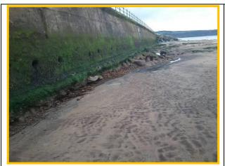
Undermining of toe in section with no rock armour **Photo from 2012.**(Asset Ref. 1221D901D0802C01)
