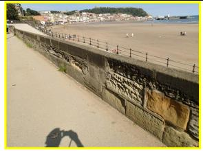
Erosion and weathering to limestone blocks in crest wall
