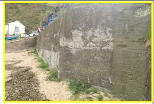
Cracking and surface damage to wall west of harbour office. (Asset Ref. 1221D901D0403C01)
