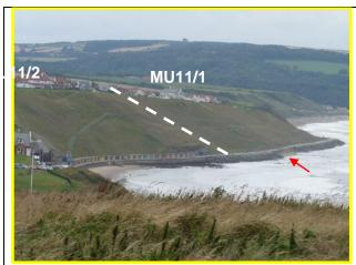
**MU11/1** Locally Active. Arrow indicates gap in rock armour and location of lower slope failures. August 2014.
