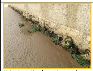
Undermining of toe of concrete encased section at bend where West Pier narrows (Asset Ref. 1221D901D1301C07)
