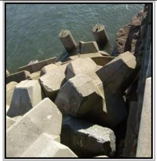
South end of harbour arm showing potential lack of armour fill **photo from 2009** (Asset Ref. 1221D901D1301C01)
