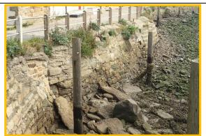
Missing pointing and voids in wall and displacement of toe armour. (Asset Ref. 1221D901D0402C06)
