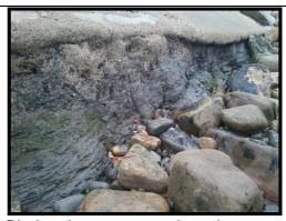
Displaced toe armour, undercutting to concrete revetment and abrasion damage to revetment. Photo from 2012 report. (Asset Ref No.1221D901D0701C02)
