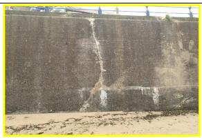
Recent repairs to vertical crack through rear harbour wall (Asset Ref. 1221D901D0403C01)
