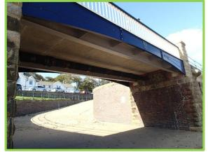
Pedestrian bridge at access slipway from Cargate Hill has been replaced. Open joints in slipway blocks need attention. (Asset Ref. 1221D901D1602C08)
