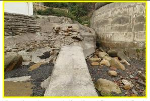
View of northern end of wall and Runswick Beck outfall with cracked concrete bagwork. (Asset Ref. 1221D901D0601C06)
