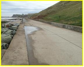
Promenade looking south east showing cracks in slabs and standing water **Photo from 2014**, **(compare to 2012 photo left)** (Asset Ref. 1221D901D0801C01)
