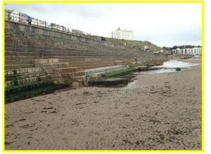
Overview photo looking north showing repairs to lower blocks and standing water in scour hole at defence toe. 26/09/2014.
