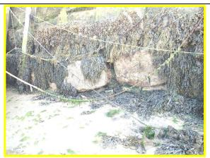
Open joints and voids between blocks in inner face of east Pier below repaired section.
