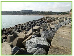
Tightly packed rock armour, Accropodes rock toe blanket and concrete toe piles seaward of East Pier harbour wall (Asset Ref. 1221D901D1301C01)
