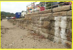
Low masonry wall at east Row Beck, north bank. Damage including missing blocks and mortar adjacent to beach shop.
