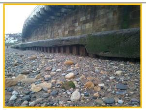
Exposure of toe piling below masonry wall. **Photo from 2012**. (Asset Ref. 1221D901D0702C04)
