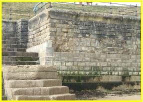
Repairs to lower blockwork on outbuilt section, upper section still to be repaired.
