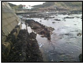
Exposed toe at Sea Life Centre. Note missing infill apron behind end of sheet pile toe. **Photo from 2012** (Asset Ref. 1221D901D1201C02)
