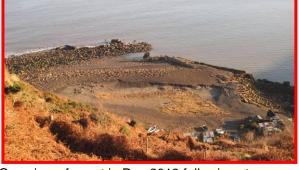
Overview of asset in Dec 2013 following storm surge of 5<sup>th</sup> Dec 2013. Significant loss of fill material adjacent to the breakwaters since July 2013 (left). (Asset Ref. 1221D901D0502C01)
