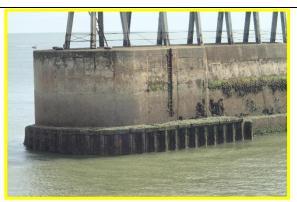
North end of outer east breakwater extension arm on 25/09/2014, showing corroded toe piles. (Asset Ref. 1221D901D0803C04)
