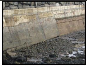
Undercutting to landward facing of north breakwater (photo from 2009 inspection) (Asset Ref. 1221D901D0402C01)
