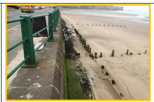
Derelict groynes and timber toe breastwork partly covered due to high beach levels. Ref. 1221D901D0702C01)
