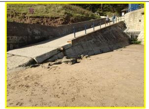
Ramp at south end of wall showing cracking in side wall and lower section of handrails missing. (Asset Ref. 1221D901D1602C05)
