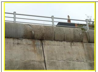
Quarter Deck sea wall with cracked capping beam with previous repairs (Asset Ref. 1221D901D1003C10)
