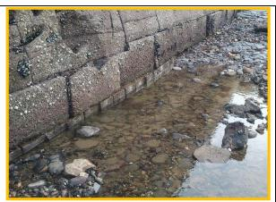
Exposed timber foundation under inner face of east breakwater **photo from 2012**. (Asset Ref. 1221D901D0803C03)
