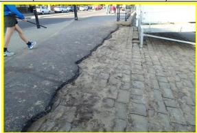
Damage at edge of road and open joints in some of the beach access ramp blockwork.
