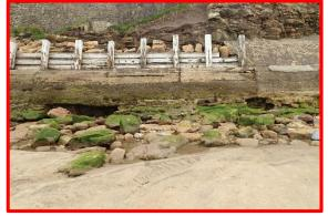
Defence toe undermined with large voids (very poor condition) (Asset Refs. 1221D901D0802C05)
