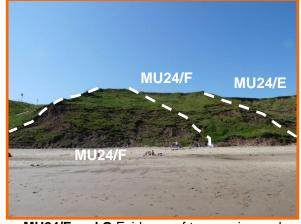
MU24/F and G Evidence of toe erosion and significant movement in lower part of slope (Partly Active). August 2014.
