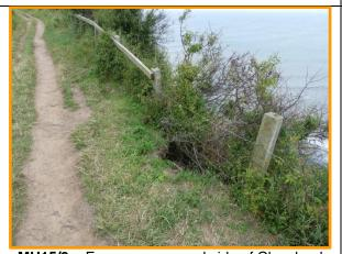
**MU15/3** – Fence on seaward side of Cleveland Way being undermined by recession of the cliff top. August 2014.
