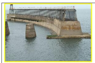
General view of outer east breakwater extension arm, on 12/09/2014 showing south end of outer east breakwater extension arm, where failed toe piling was replaced with precast concrete panels in 2012. (Asset Ref. 1221D901D0803C04)
