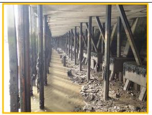
View under west quay, with original wall on right, showing corroded deck support piles Asset Ref. 1221D901D0803C06
