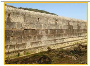
Undermining of wall, with voids at South Bay Pool (Asset Ref. 1221D901D1303C02)
