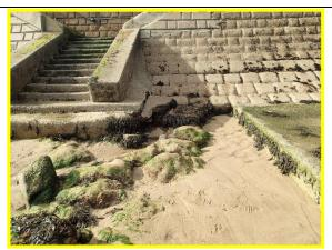
Erosion and undermining at central steps at south end of Asset Ref. 1221D901D1201C07
