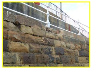
Cracking, mortar loss, damage to capping (Asset Ref. 1221D901D0802C07)
