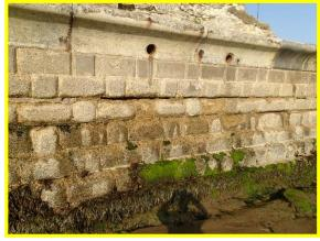
Area of washed out joints, abrasion and undercutting. (Asset Ref. 1221D901D1302C02)
