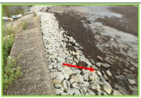
Section of rock armour with gaps / displaced units in front of 2001 seawall. (Asset Ref. 1221D901D1003C01)
