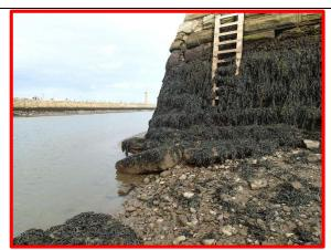
Toe undermining and erosion damage at seaward end of Tate Hill (old RNLI) pier. (Asset Ref. 1221D901D0803C08)
