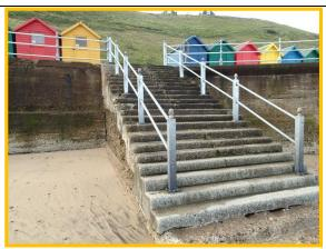
No change from 2009 to stair sidewalls, but new handrails. (Asset Ref. 1221D901D0802C04)
