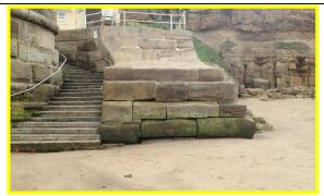
Evidence of repairs and repointing to upper blocks (Asset Ref. 1221D901D0802C12)
