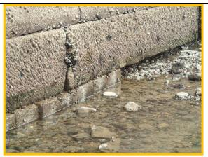
Exposed timber foundation under inner face of east breakwater **photo from 25/09/2014**. (Asset Ref. 1221D901D0803C03)
