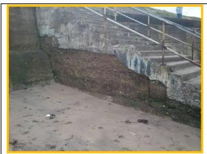
Erosion and cracking to stair side wall - **Photo** from 2012 (Asset Ref. 1221D901D0802C04)
