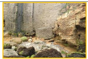
Example of undercutting at interface with cliff requires repair -poor condition.
