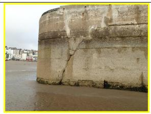
Cracks and repairs in concrete encasement section at narrowing of West Pier (Asset Ref. 1221D901D1301C07)
