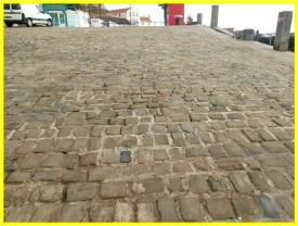
Washout of mortar in masonry blocks on harbour access ramp (Asset Ref. 1221D901D1301C11)
