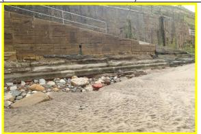
Undermining of toe and damaged blocks(Asset Ref. 1221D901D0802C06)
