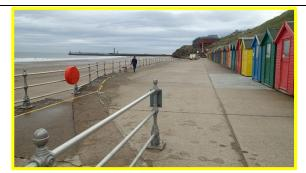
General view of promenade showing new handrails, repaired slab, and open joints. (Asset ref. 1221D901D0802C14)
