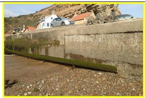
Cracks in wall adjacent to slipway (Asset Ref. 1221D901D0402C03)
