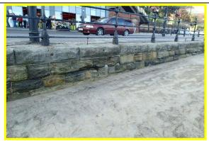
Damaged blocks and washed out joints needing repair. (Asset Ref. 1221D901D1301C24)
