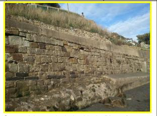
Gaps at joints and missing blocks **Photo from 2012** (Asset Ref. 1221D901D0601C03)
