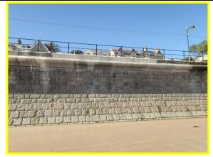
View of wall showing repaired coping and wave return blocks and abrasion damage to blocks near beach level. (Asset Ref. 1221D901D1602C08)
