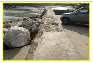
Surface erosion and exposed aggregate to southern end of promenade.
