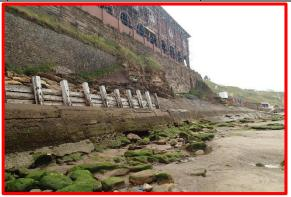
Weathering and loss of cliff material above failed toe protection (Asset Ref. 1221D901D0802C05)
