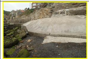
Repaired vertical cracks to toe of wall, and horizontal cracks holding (Asset Ref. 1221D901D0601C06)
