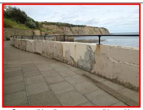
Crest wall locally very poor condition, with evidence of recent cosmetic repairs.
