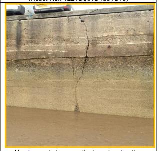
No change to large vertical crack extending through the wall, but beach levels higher than in 20012 or 2009. **Photo 10/09/2014** (Asset Ref. 1221D901D1301C19)
