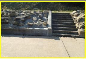
Grouted revetment behind prom has been repaired in many locations Asset Refs. 1221D901D1201C25 & C04
