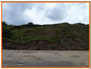
**MU29/AB** Eroding toe and sliding mid-slope (Partly Active). August 2014.
