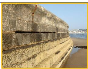
Repaired upper section of upper wall adjacent to re-constructed concrete ramp.
