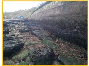
Undermining of toe in section with no rock armour **Photo from 2012.**(Asset Ref. 1221D901D0802C03)
