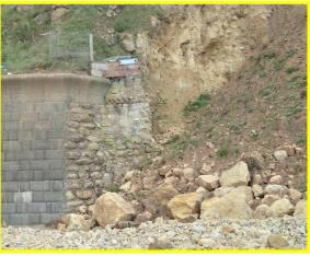
Tie in of Pumping station defences at north end note erosion of cliff compared to photo on left.
