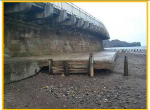
Masonry blockwork sea wall with cantilevered footway, showing large void under toe apron and failed groynes. **Photo from 2012.** (Asset Ref. 1221D901D0702C04)
