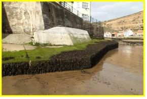
Additional section of toe berm placed since 2012 to stabilise wall (Asset Ref. 1221D901D0403C05)
