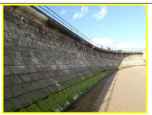
General view of wall showing area of damaged blocks and previous repairs to coping / splash beam. (Asset ref. 1221D901D1602C07)
