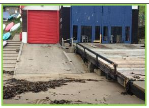
The timber slipway at the old RNLI building has been repaired. (Asset Ref. 1221D901D0601C04)
