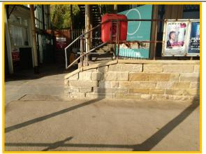
Weathering and loss of joints in stone wall at back of high level prom by cliff railway (Asset Ref. 1221D901D1302C01)
