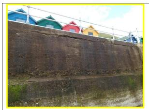
Horizontal cracks in wall (Asset Ref. 1221D901D0802C04)
