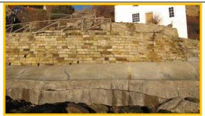
Toe of cottage wall, 17th December 2013. Note loss of timber fencing and undercutting of toe due to December 2013 storm event. (Asset Ref. 1221D901D0601C06)
