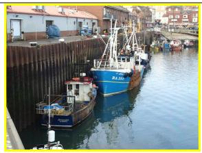
Corroded sheet piling of West Pier (Asset Ref. 1221D901D1301C13)
