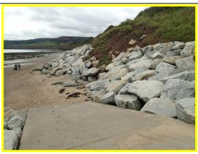
Cliff slump has partially covered and damaged the revetment. (Asset Ref. 1221D901D1003C07)
