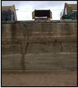
Large vertical crack extending through the wall photo from 2009
