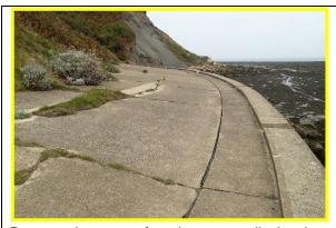
Promenade on top of northern seawall, showing movement of crest slabs and vegetation growth in damaged areas, 12/09/2014 (Asset Ref. 1221D901D0601C01)
