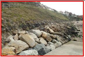
Displaced rock armour and damaged revetment at the Haggerlythe inside harbour adjacent to East pier (Asset Ref. 1221D901D0803C05)
