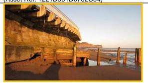
Photo from 17th December 2013, showing larger void under toe apron and failed groynes. (Asset Ref. 1221D901D0702C04)
