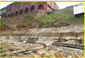
**MU11/3** – Failure of both till slope and exposed rocks above defences. August 2014.
