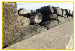
Missing crest armour unit on the north breakwater at approx. 1/3 way along crest (Asset Ref. 1221D901D0402C01/2)
