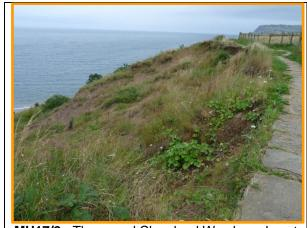
**MU17/2** - The paved Cleveland Way has almost been undermined by recession of the cliff top. (Partly Active). August 2014.
