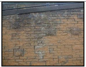
Vertical crack to second wall protecting road. **Photo from 2009** (Asset Ref.
