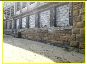
Abraded and spalling concrete capping to original wall below in filled openings (Asset Ref. 1221D901D1301C29)
