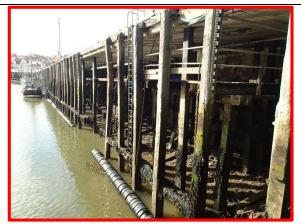
Broken and missing timber fender piles at fuel berth need replacing urgently to protect the deck support piles. Asset Ref. 1221D901D0803C06)
