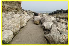
Storm damage displaced armour stones near root of north breakwater
