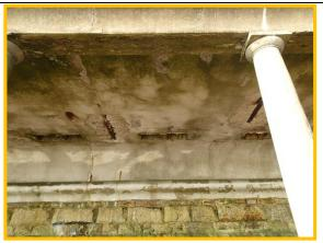
Cracking and corrosion to beams and upper level deck slab
