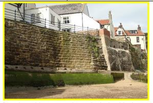
Repairs evident to cracks and missing blocks replaced, but repairs continue to be required. (Asset Ref. 11221D901D0402C22)
