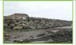
South breakwater outer face rock armour in good condition. (Asset Ref. 1221D901D0403C03)
