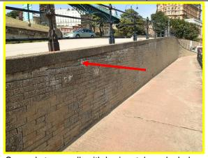
Second stage wall, with horizontal cracks below coping, 10/09/14
