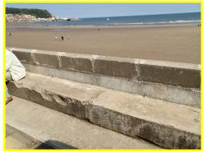
Parapet wall has been rebuilt following December 2013 storm, but crest wall needs constant attention to repairs. (Asset Ref. 1221D901D1301C27)
