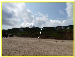
**MU29/**E2 and EF – Units immediately north of Hunmanby Gap. Erosion is taking place at the toe but is much less evident in the upper cliff than in the units immediately to the north. August 2014.
