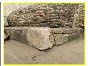
Wide cracks to toe of wall and undermining (Asset Ref. 1221D901D1003C06)
