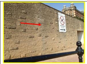
Second stage wall, with vertical crack, 10/09/14 (Asset Ref. 1221D901D1301C09)
