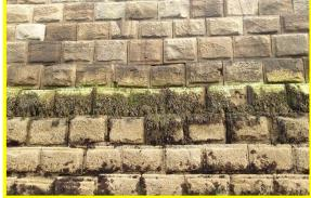
Displacement of block work on west side of West Breakwater - left image from 2009, right from 12/09/14 (Asset Ref. 1221D901D0803C02)
