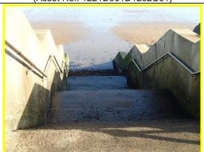
Scour hole at toe of steps prevents use at low tide. Note abraded / corroded steps.
