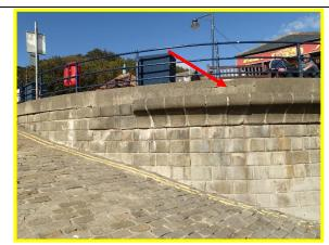
Cracks in coping and damaged blocks at ramp with evidence of previous repairs. (Asset ref. 1221D901D1602C06)
