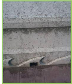
Example of crack through centre of wave wall – photo from 2012 (Asset Ref. 1221D901D1202C03)
