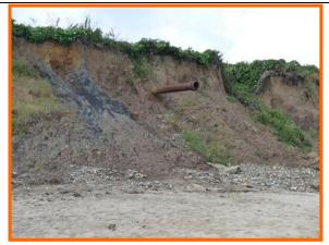
**MU29/AS** Protruding pipe illustrating ongoing erosion in this unit (Partly Active). August 2014.
