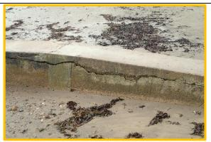
Large horizontal crack to breakwater photo from 12/09/2014 (Asset Ref. 1221D901D0601C02)
