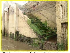
Cracks to concrete facing and exposed toe to steps on West Pier (Asset Ref. 1221D901D1301C18)
