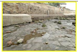
Exposed mudstone platform and undermining of wall toe 12/09/2014 (Asset Ref. 1221D901D0601C03)
