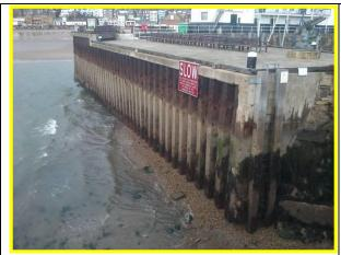
Corroded sheet piles, but overall fair condition **Photo from 2102** (Asset Ref. 1221D901D1301C17)
