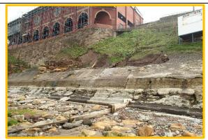
Concrete revetment toe in poor condition and slumps and failures in cliff below building. (Asset Ref. 1221D901D0802C15)
