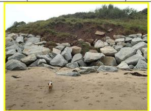
Cliff slump has partially covered and damaged the revetment. (Asset Ref. 1221D901D1003C07)
