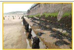
Condition of wall, which was rated as poor in 2012 is similar or worse despite higher beach levels. (Asset Ref. 1221D901D0702C01)
