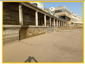
Repairs have been undertaken to lower level wall, but defence remains in poor overall condition (Asset Ref. 1221D901D1302C01)
